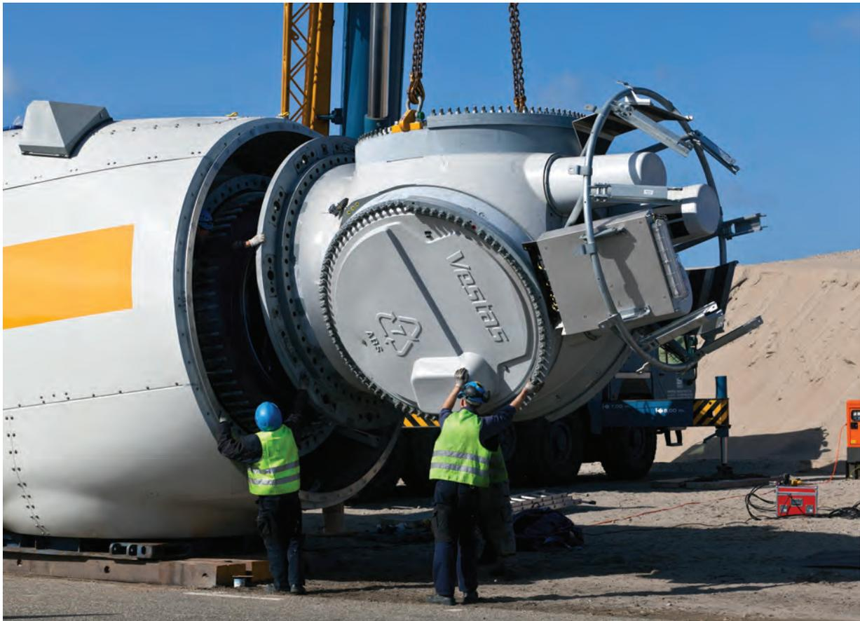
At a wind turbine construction site, workers mount the rotor hub onto a turbine gearbox or generator.
