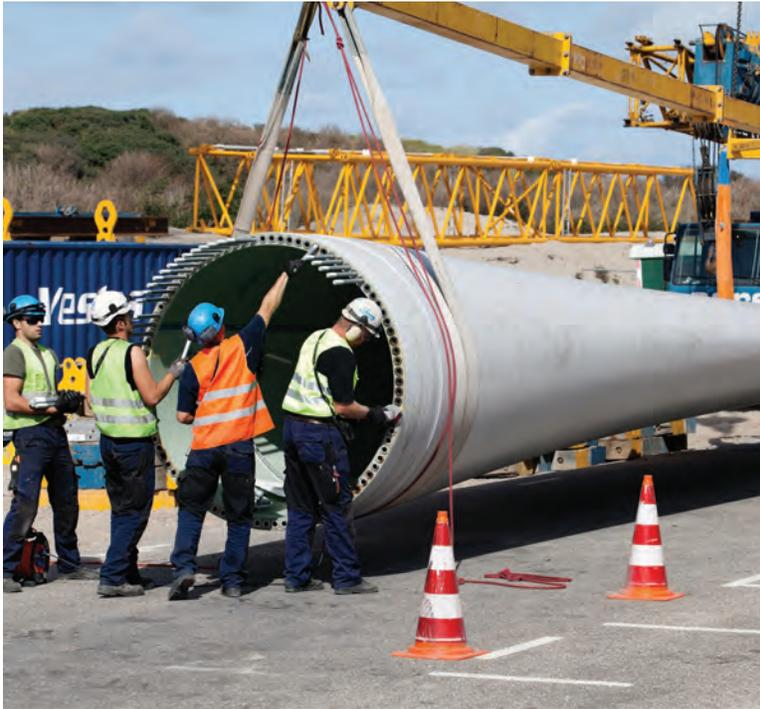
Construction workers install bolts in the shaft end of a wind turbine blade.
